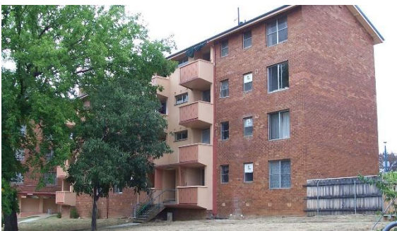
Stuart Flats, in Light Street, Griffith, ACT. They were owned by Housing ACT. The flats were demolished in October 2019.
